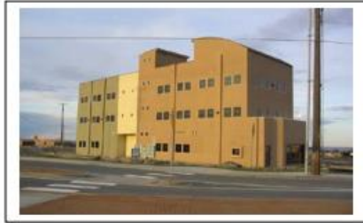
Lack of adequate façade transparency fails to create an indoor-outdoor relationship.
